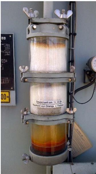
Moreover, in the conventional dehumidifier, the oil is also entered through the oil reservoir into the silica gel. The negative impact of the oil is often clearly visible. The lack of cleaning the outflowing air and additionally attached exposure to the oil reservoir, the silica gel is contaminated from both sides. The drying of the air is thus limited, and the moisture in the transformer rises
