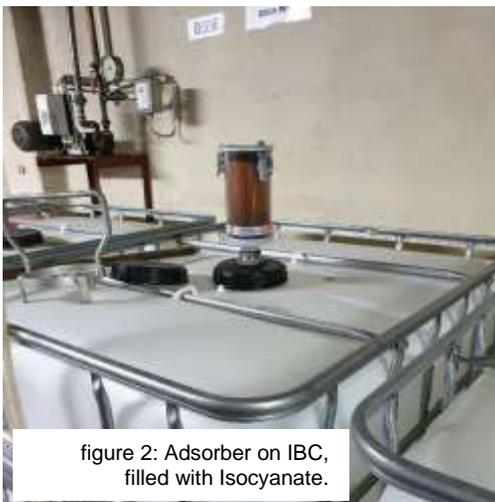
figure 2: Adsorber on IBC, filled with Isocyanate.
