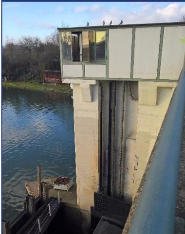
There are two gears in each weir. These regulate the water level depending on the weather. By raising and lowering the single or upper guard, the gears are set in motion every hour.
