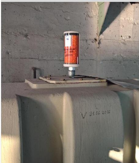
Breathable dryers are indispensable for protecting the gear units on weirs from condensation damage. Through the use of adsorbers, the humidity in the gearbox is reduced and the dew point (temperature at which the air liquefies) is lowered to high minus degrees.
